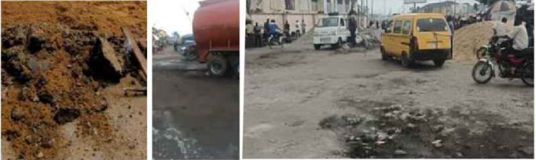
MOBIL ROAD (undergoing repairs)
